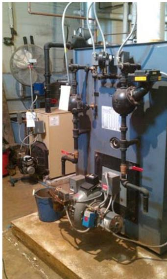
Engineers expect to upgrade the heating system on all three floors of the Franco-American Heritage Center. The upgrade includes converting the larger steam boiler to hot water and converting the entire system from oil to gas. According to the engineers the steam-to-hot water conversion should result in an immediate 25 percent energy savings. The smaller boiler will be removed. The larger boiler has sufficient capacity to heat the entire building.
